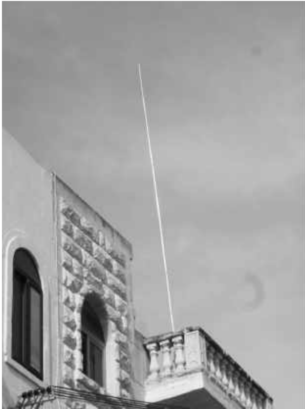
A view of our low band vertical from street level
